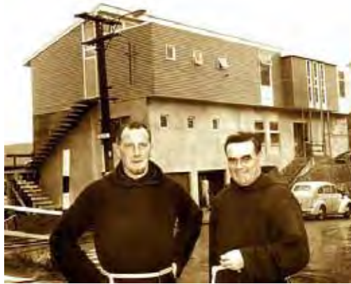
Brothers Matthias and Agathangelus outside the newly built St Anthony's Friary at the corner of the Rigi and Glenmore St. in Kelburn
